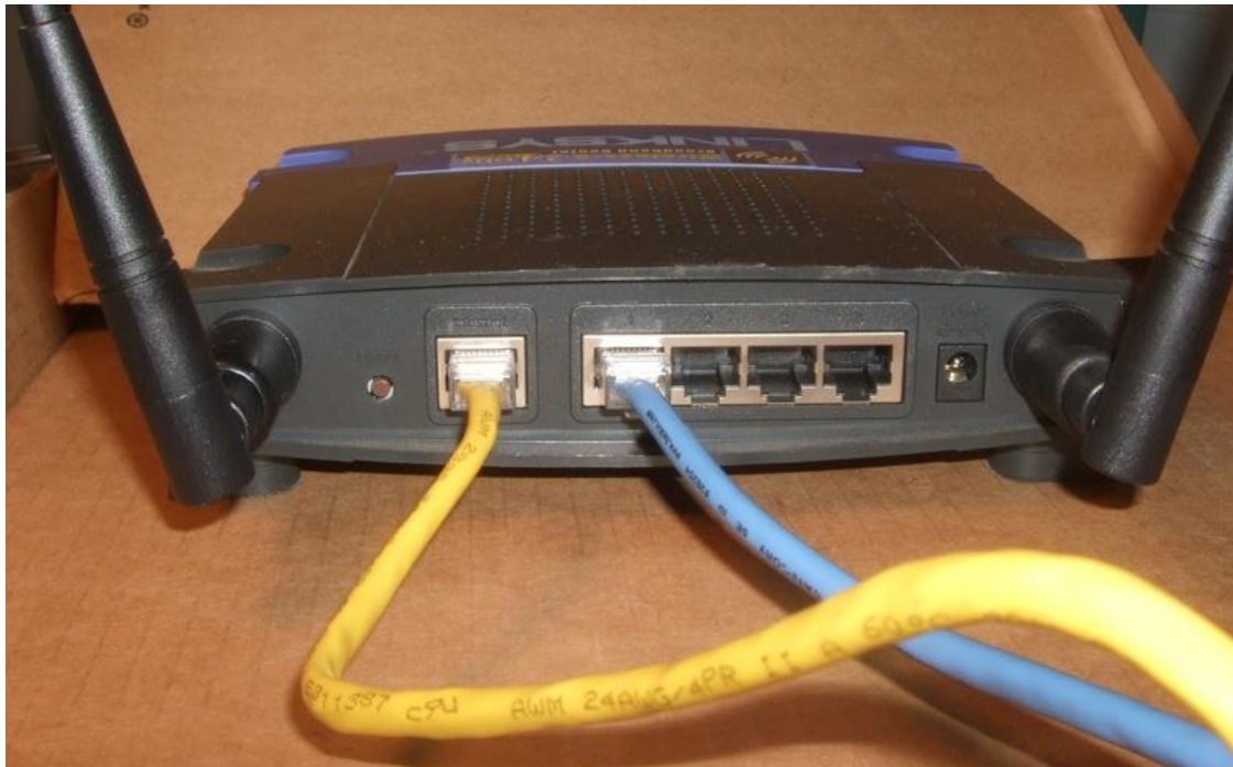
Ethernet cables plugged into the back of a Wi-Fi router
